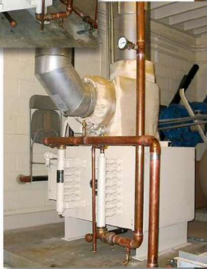
HRSR-116826.5ALS (above) Murrieta High School, Murrieta, California Recovering Exhaust Heat from a natural gas 60kW micro turbine; cooling 856 SCFM from 580°F to 289°F; and heating 40 GPM of water from 75°F to 90.2°F.
