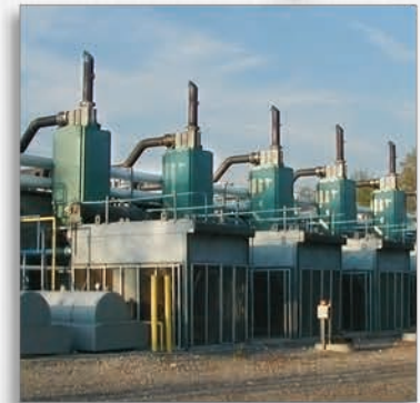
Innovative Energy Systems , Oakfield, New York (7) Model HRSR-330C26SSP Recovering 1,845,000 Btu/hr each from (7) Caterpillar 3516 engine. Reducing each 922°F to 387°F @ 2,766 SCFM; Raising 300 GPM hot water from 180°F to 194°F.
