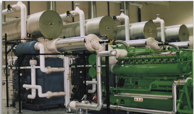
Hospital , Renton, Washington (4) Model ESG1-616B19CSS Recovering Btu from (4) Jenbacher JMS-320, 900kW natural gas engines. Reducing each 2,498 SCFM from 977°F to 392°F. Delivering 1,863 pph steam @ 90 PSI operating (150 PSIG design).
