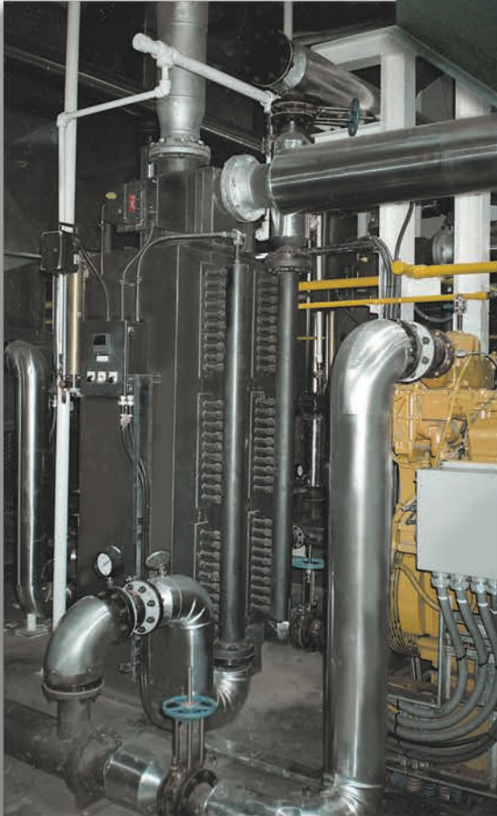
Hospital, Ontario (2) Model HRSR-336B28CSS Recovering Btu from (2) Cummins Wartsilä CW180, natural gas engines. Reducing each 968°F @ 3,666 SCFM to 339°F. Raising 175 GPM hot water from 195°F to 229°F.
