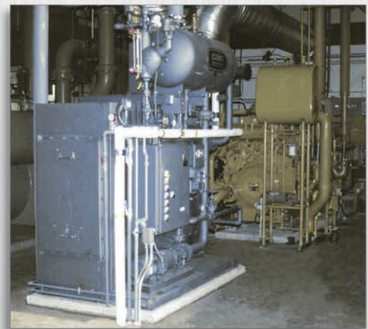
Water Purification Plant , Burlington, Ontario Model ESG1-A12D18CSS Recovering Btu from a Caterpillar 3516, 800kW natural gas engine. Reducing 2,382 SCFM from 770°F to 344°F. Delivering 1,277 pph steam @ 130 PSI operating (150 PSIG design).
